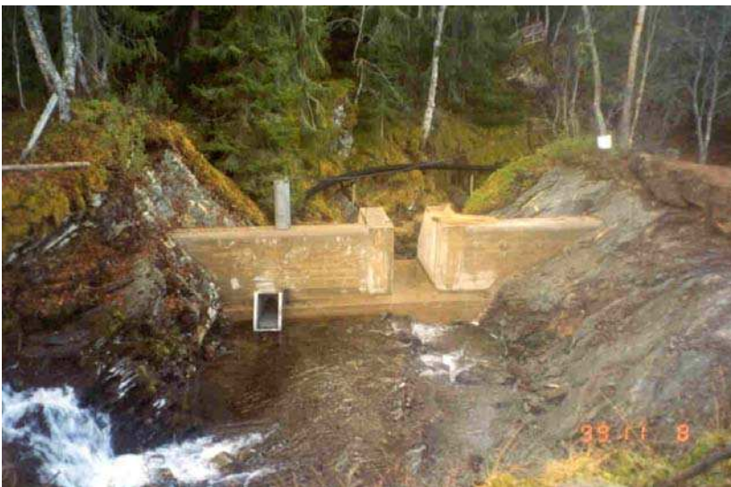
Figure 3.1.4. 2: Intake dam at Glisja power plant in the municipality of Midtre Gauldal
