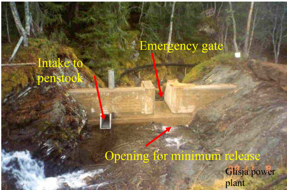
Figure 3.1.1.9. Dam to Glisja power plant in Soknedal
